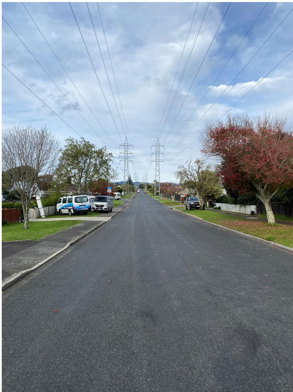
Photo 1 – Powerco assets and Transpower assets on Pooles Road, Greerton, Tauranga
