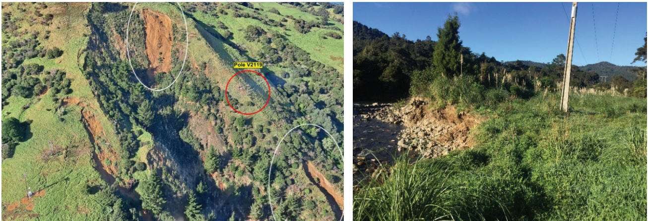
Figure 11 – During Cyclone Gabrielle, slips and trees damaged the network and put assets at risk. The slips undermined key circuits in the Coromandel, up the coast in Colville, and river scouring put nearby subtransmission structures at risk of collapse, right.
