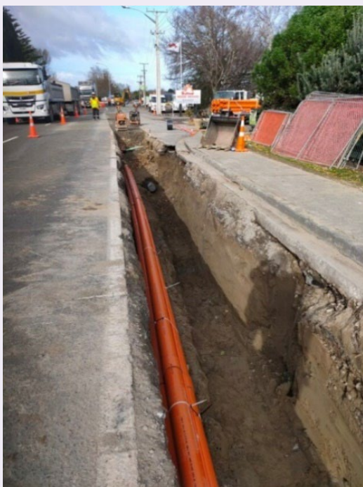
Figure 44 – New 33kV cable near Bulls substation, left, and new Ohakea substation, right.
