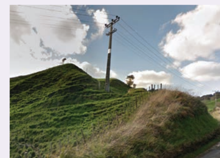
Figure 34 – Supply to Whanganui from Brunswick GXP travels through an area of active slips. We are reviewing this line for potential land movement.
