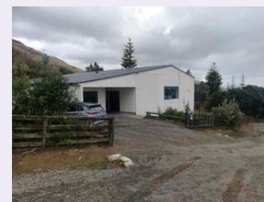
Figure 45 – We are working with the community at Ākitio on potential backup supply options.
